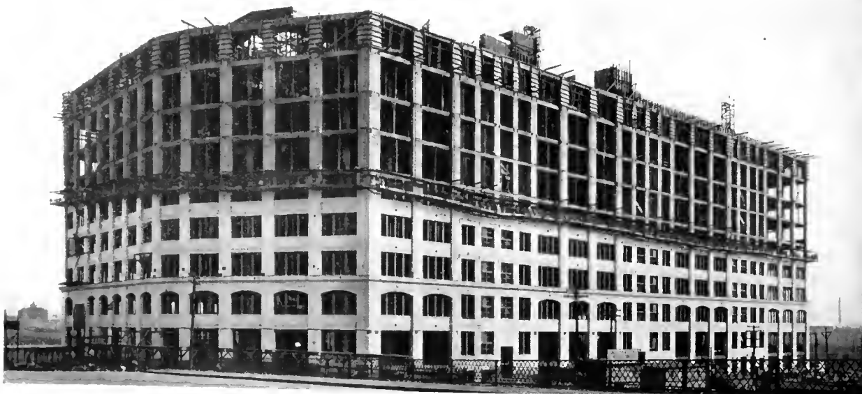
PROGRESS VIEW Illustrating method of carrying up terra cotta facing
